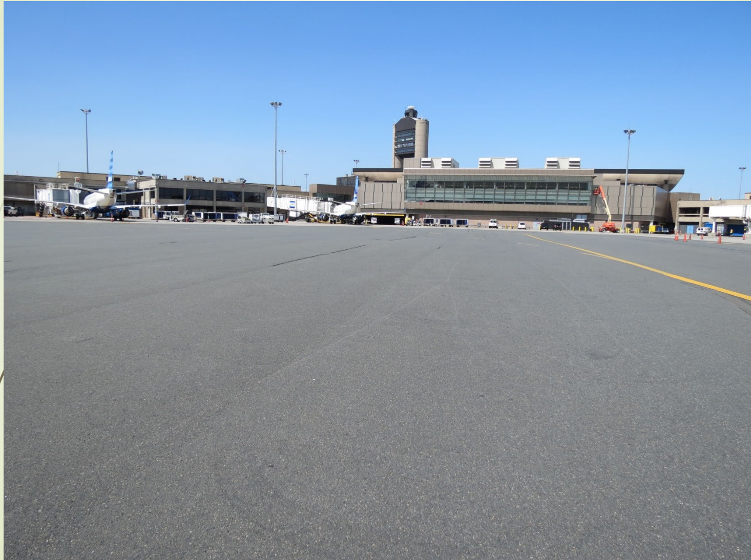
9 year old FR Alleyway Pavement
